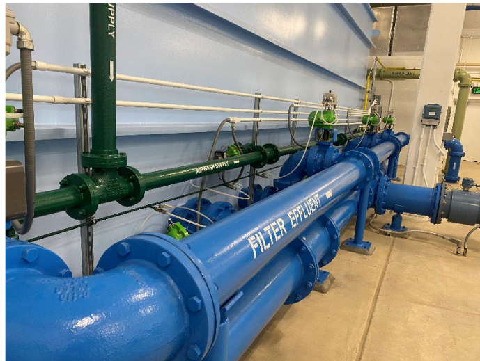
City of Appleton Construction of a New Drinking Water Treatment Plant
